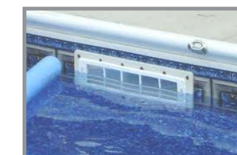
There are very inexpensive safety face plates that can make the skimmer harder for hands to reach.
